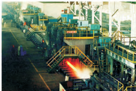
24-stand Continuous Rolling Mill(POMINI)
