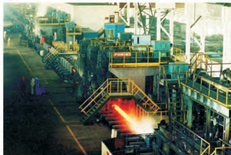
24-stand Continuous Rolling Mill (POMINI)
